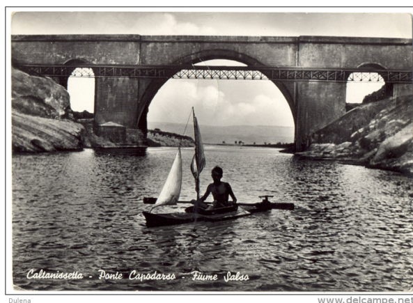
FIGURE 4 – A 1950s picture of Salso River, Capodarso Bridge.
